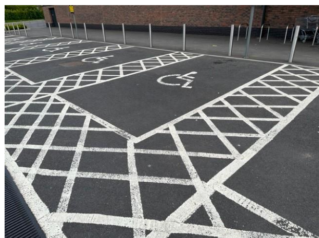
Disabled parking with additional width provided on both sides and the rear. Access to the footway to the front of the spaces is level.
