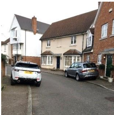
Footway parking creates obstructions for pedestrians and can cause safety concerns.
